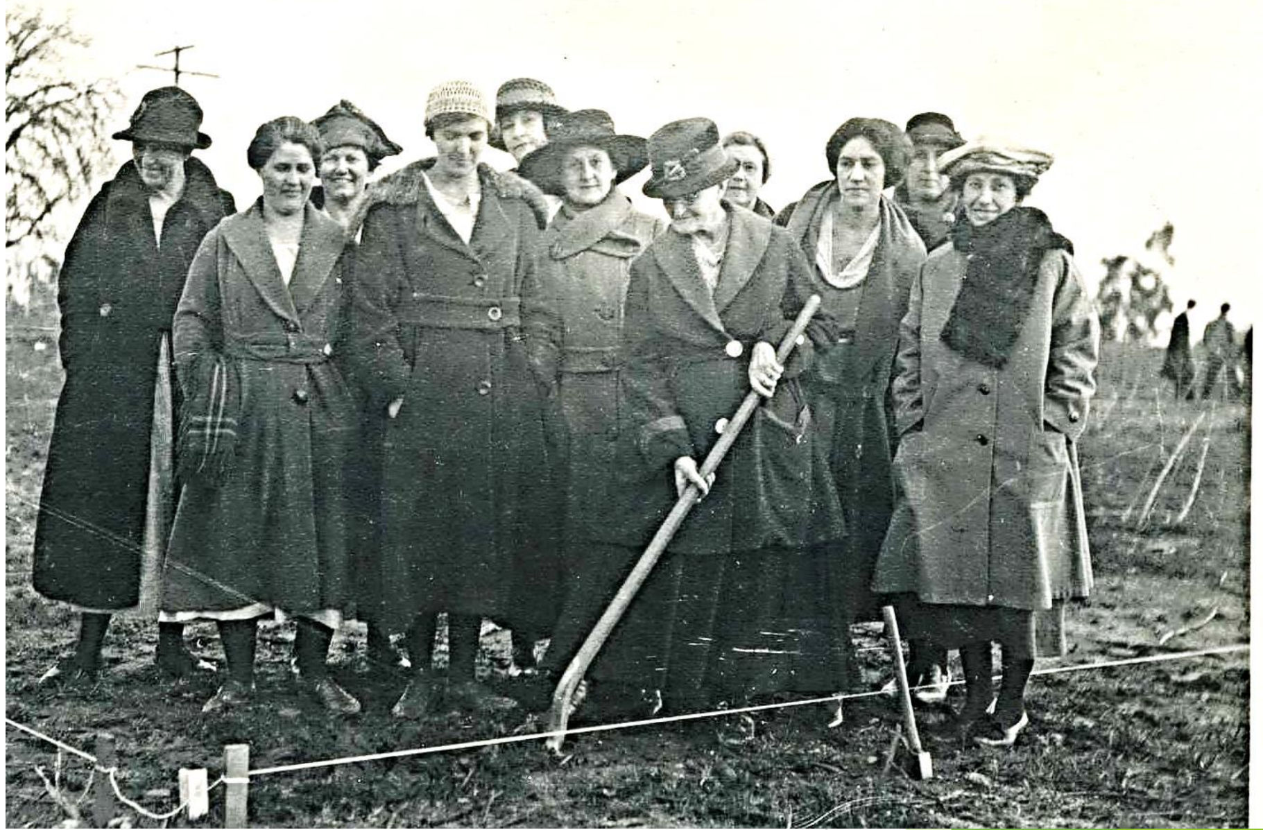
Breaking Ground for the Club Building
